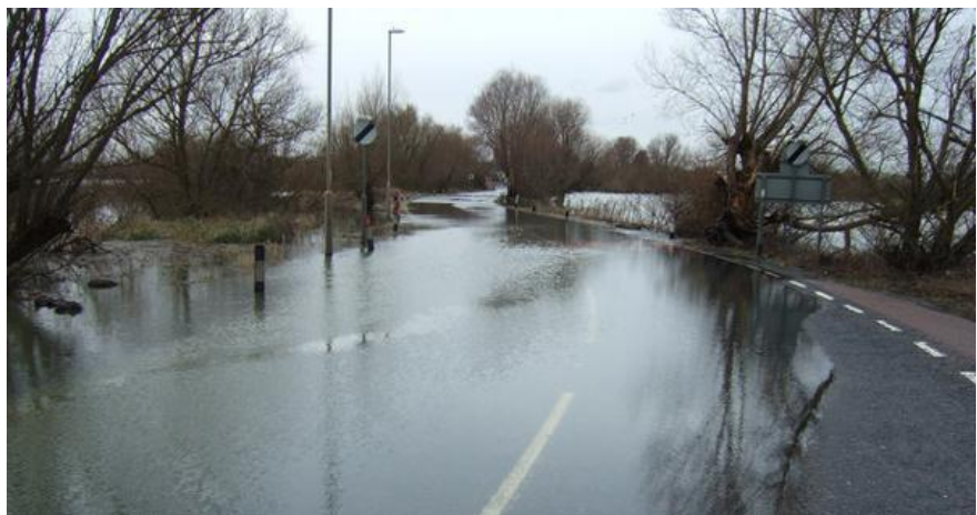
Flooding on the A1123 at Earith
