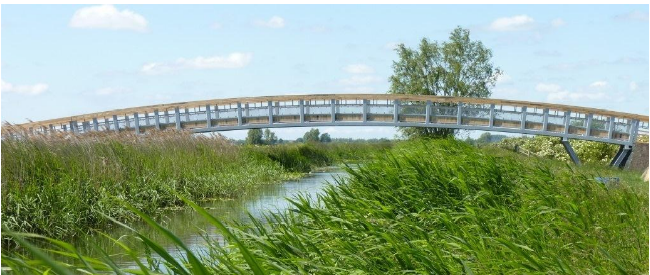
Reach Lode pedestrian and cycle bridge taking National Cycle Network Route 11 between Wicken Fen and Anglesey Abbey
