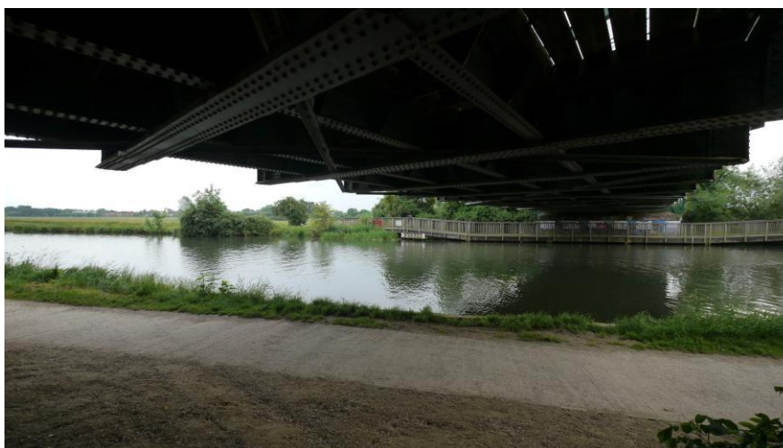
The cycle bridge over the River Cam will be located to the east of the railway bridge, and will link to the Haling Way and Cambridge to Newmarket cycle routes on either side of the river.
