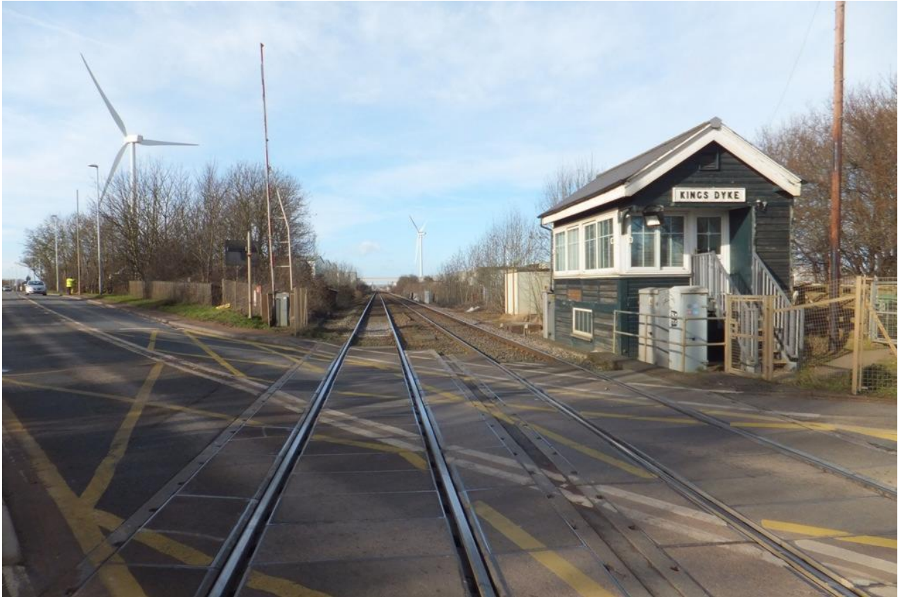
The Kings Dyke level crossing
