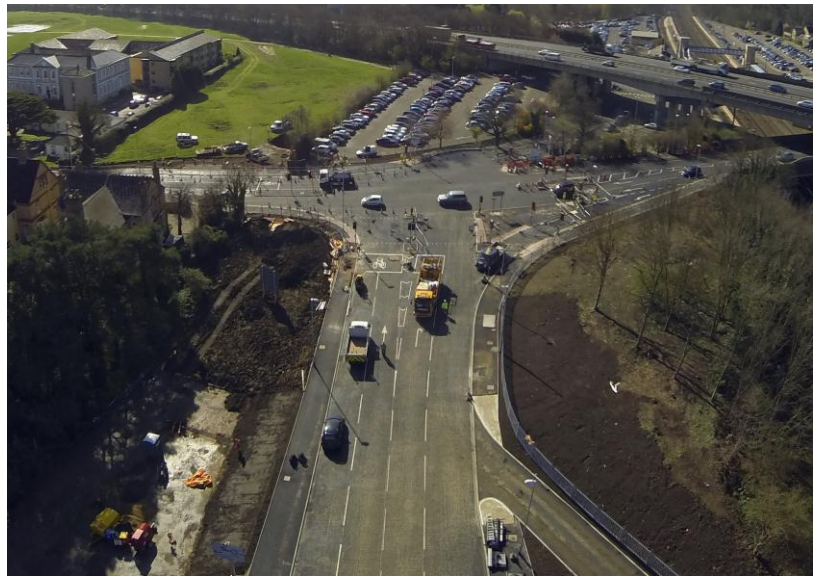
The junction of Brampton Road with Huntingdon Station access and the new Huntingdon West of Town Centre Link Road (Edison Bell Way), which is opening up land for development.
