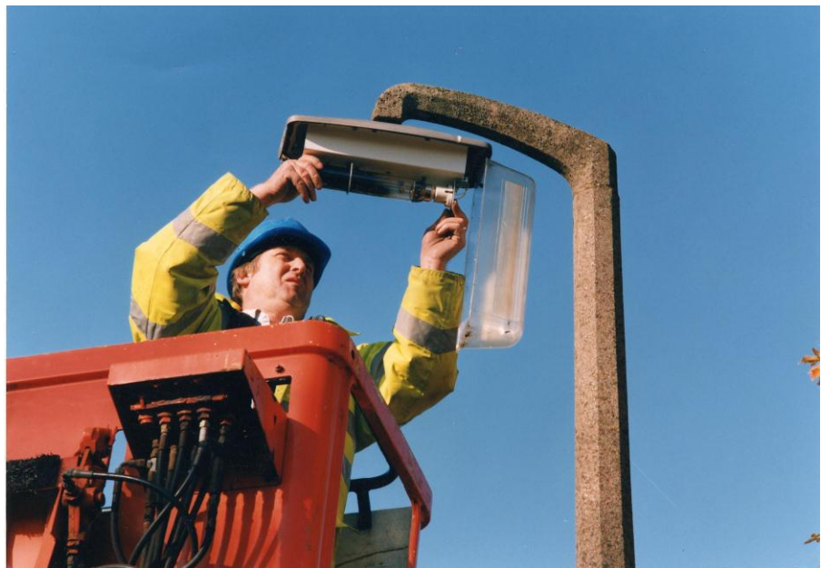
Street light maintenance
