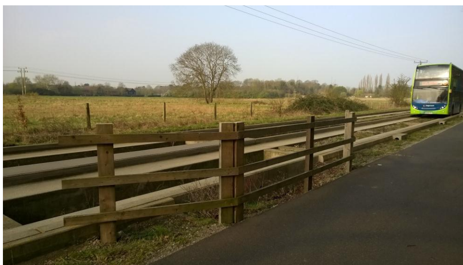
Tunnel for toads under the Busway at Histon
