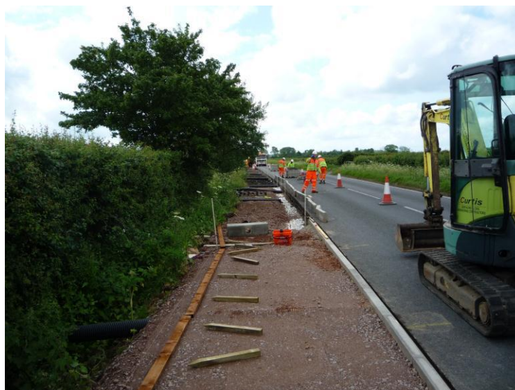
Construction of the Swavesey to Buckingway Business Park cycle route
