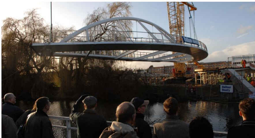
The Riverside Bridge in Cambridge, which was part funded by development
